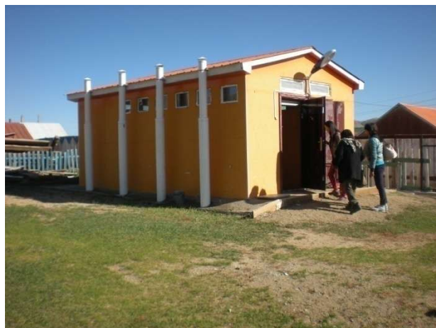
New VIP latrine in Galt school
