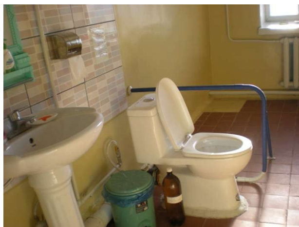
Rehabilitated indoor WASH room in Tarialan dormitory
