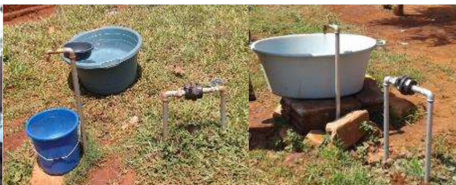
Photo 9: operational stand post in Espungabera Photo 10: private connections in Espungabera
