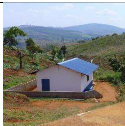
After the rehabilitation
