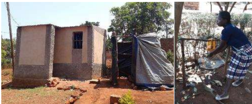
Photo 13: New latrines on the left, old latrines on the right Photo 14: Tippy taps
