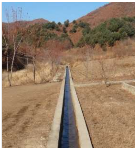
Low Water Flow from Catchment, Unsan County
