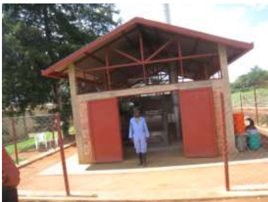
Figure 3: High temperature incinerator in Kanombe
