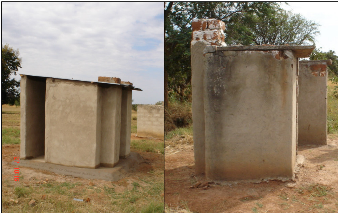
(a) Iron-roofed VIP latrine
