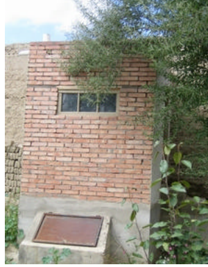
Elevated dry composting latrine; the opening at the back provides for the removal of the digested sludge for use as organic fertilizer
