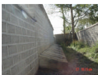
Dry composting pit openings at the back of the latrine building
