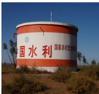
Ground water is pumped to this storage tank to provide piped water by gravity to a newly built herders' resettlement colony
