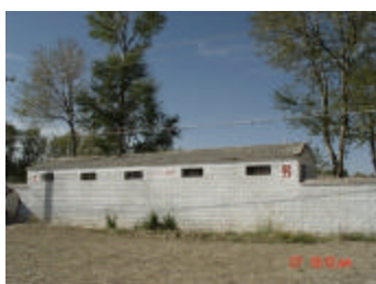
A primary school sanitary latrine building (dry composting type)
