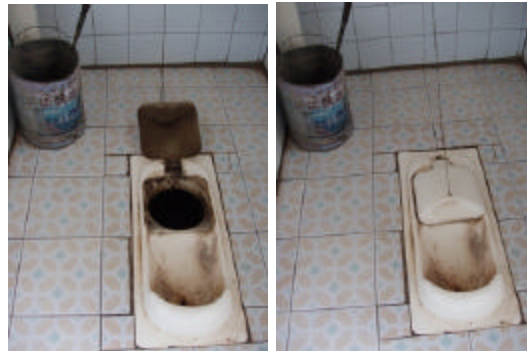
The squatting pan of urine-separate sanitary latrine in an open and closed position
