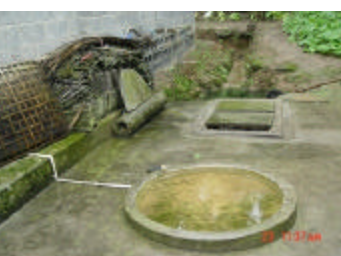
Household bio-gas plant treating human excreta and pig manure
