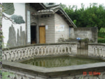
A family's water reservoir and a sanitary latrine
