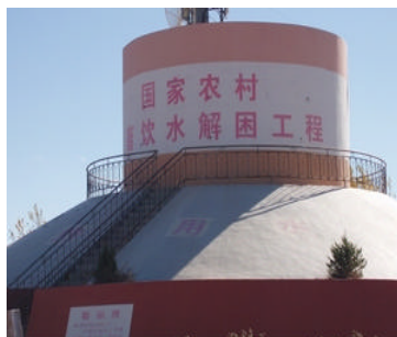
An elevated and insulated water tank providing safe water to villages, including schools
