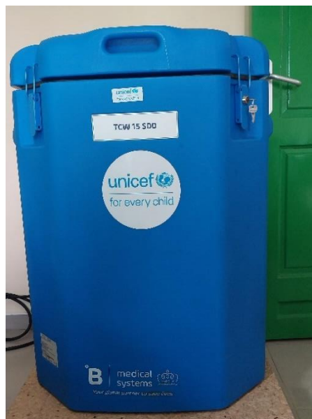
Figure 6 Solar powered refrigerator at Hekoenoenoe MM Health facility
