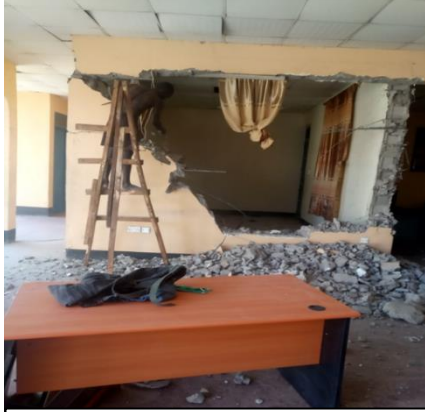
Renovations of JSWA Women's Empowerment Centre
