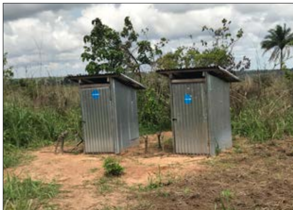
Picture 4: Latrines for a school with 400 pupils
