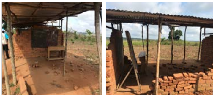
Pictures 7 and 8: Examples of semi-permanent rehabilitation
